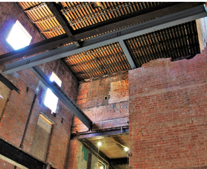
Preserving the original front doors and as much of the brick as possible was integrated into the design of Pepper's new headquarters..
